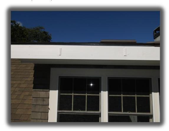
The thickness of your stand-off block is determined by the placement of the drip edge.
